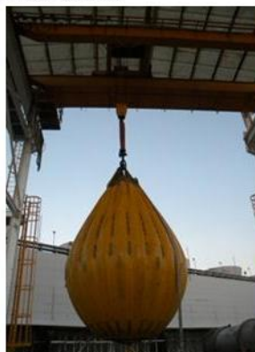
25te Pumps outdoor crane
